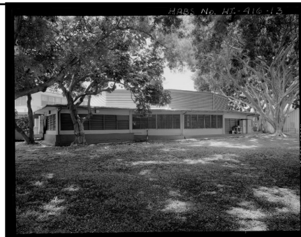
Bloch recreation center and arena
