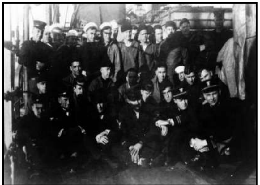
The surviving crew members of USS Jacob Jones DD-61 (See photo at right)
